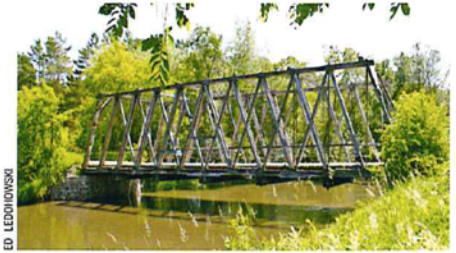
Howe Pony Timber Truss Bridge (1918)
